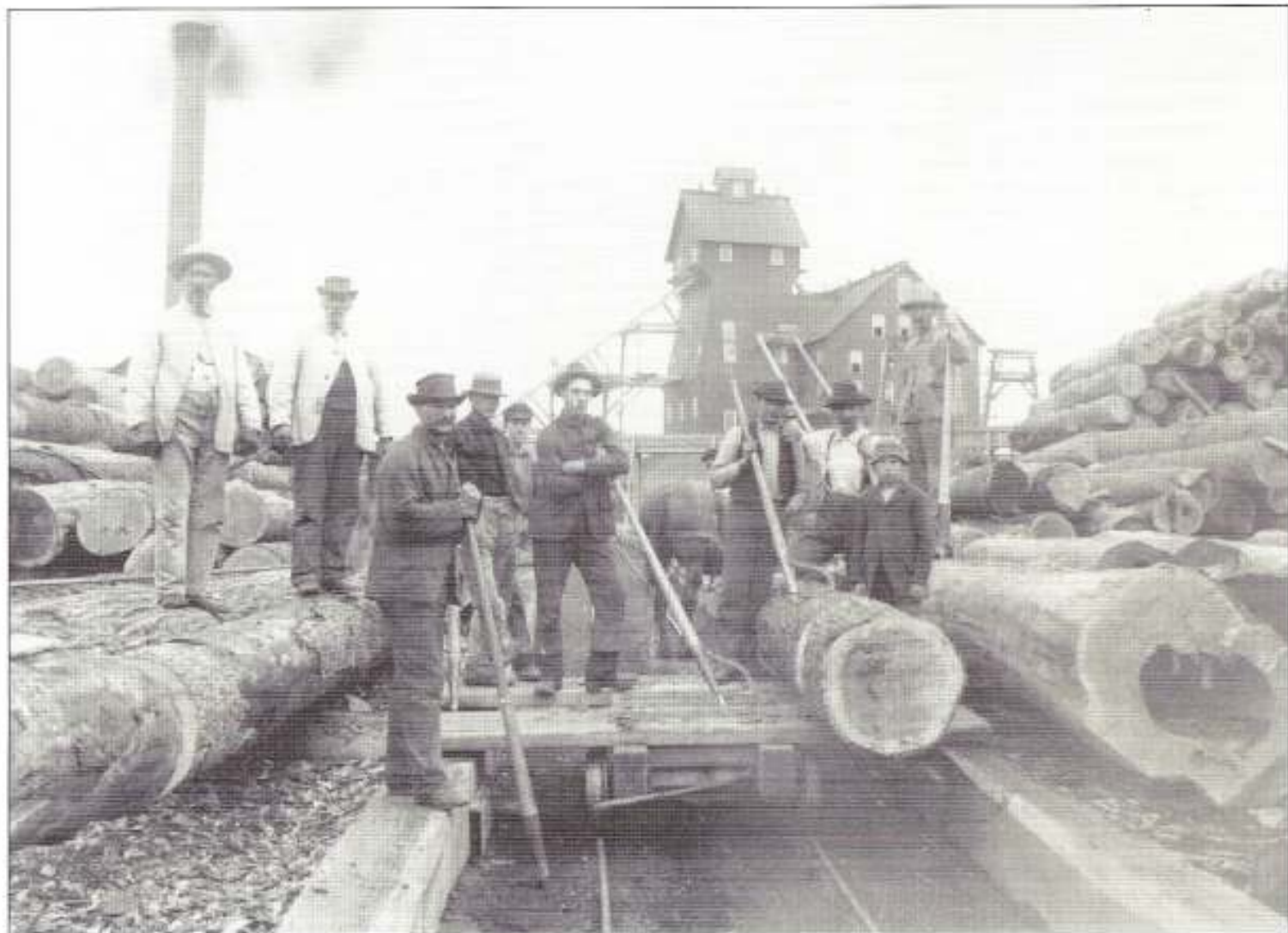
A 1903 view of the timber yard at the Tamarack #2 mine. A tremendous amount of timber was consumed for ground support in the mines. Photo by John T. Reeder.
